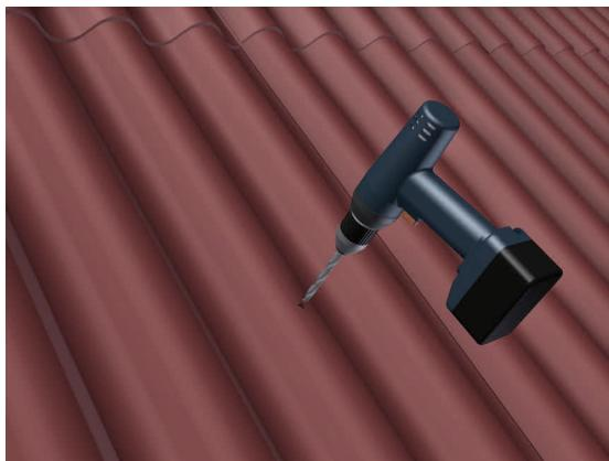
The fixing of the roof construction is done with the solar fastener with sealing. After having determined the mounting position of the solar fastener the corrugated plates must be pre-drilled centrally on the wave according to manufacturer instruction.
