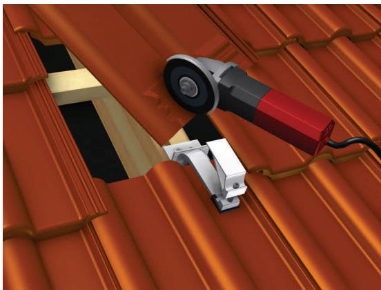
Now the removed roof pan tiles are re-inserted. In this connection in the range of the support shaft the lower bead of the pan tile will be polished by means p. e. of an angle grinder or a tile milling machine so that the pan tile lays flush.
