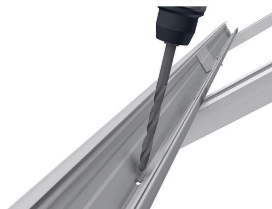
If not present or if covered at the horizontal profiles, before inserting the modules, water drainage holes must be drilled with a spacing of a module width if not present or if covered. (Ø approx. 10 mm).
